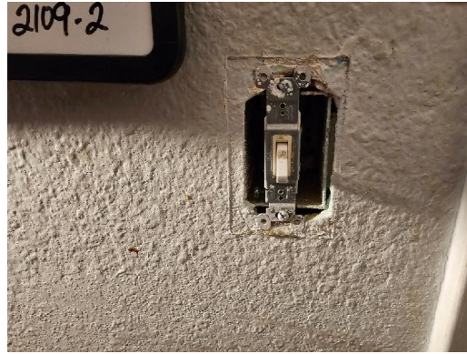
2109-2 Drywall/Joint Compound Typical Interior
