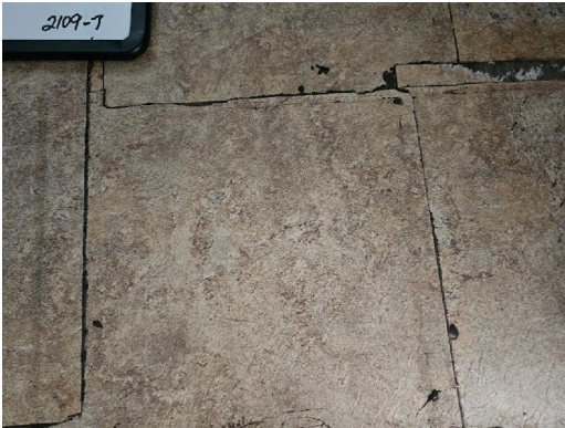
2109-7 12"x12" Floor Tile (2% Chrysotile) Typical Interior (Appx 40 sq ft)
