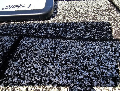
2109-1 Asphalt Shingle Typical Exterior Roof
